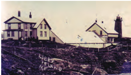
Maine's Libby Island Lighthouse in Machias Bay where Frederic W. Morong and his family lived September 6, 1895 to June 1, 1898. The only things left on the island today is the tower and fog signal building; everything else was demolished by the Coast Guard. Today the island is part of the Petit Manan National Wildlife Refuge. ( Lighthouse Digest archives.)
